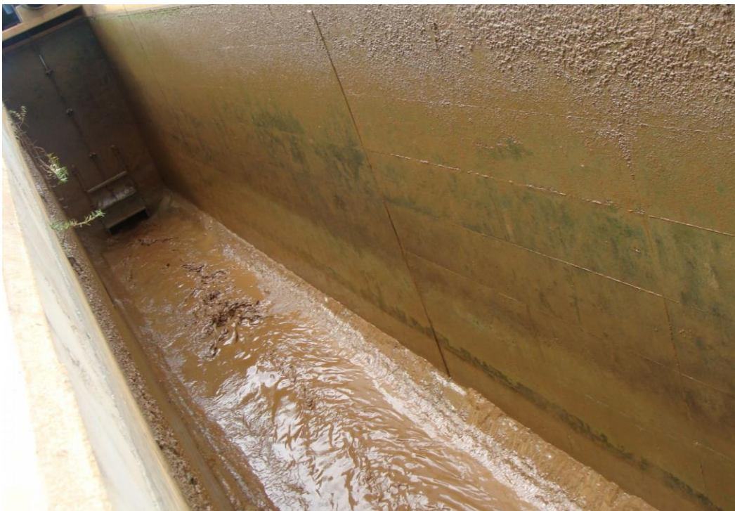
Figure 2: View of inside of desilting channel at Lebalelo Weir Desilting Works (example)
